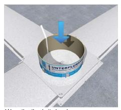
**4** | Inserting the shuttering pipe Insert shuttering pipe straight from the top into the floor box opening. Floor box and shuttering pipe make one mounting unit. Mask all openings in the duct system. Apply insulation flush to duct system and to shuttering pipe.
